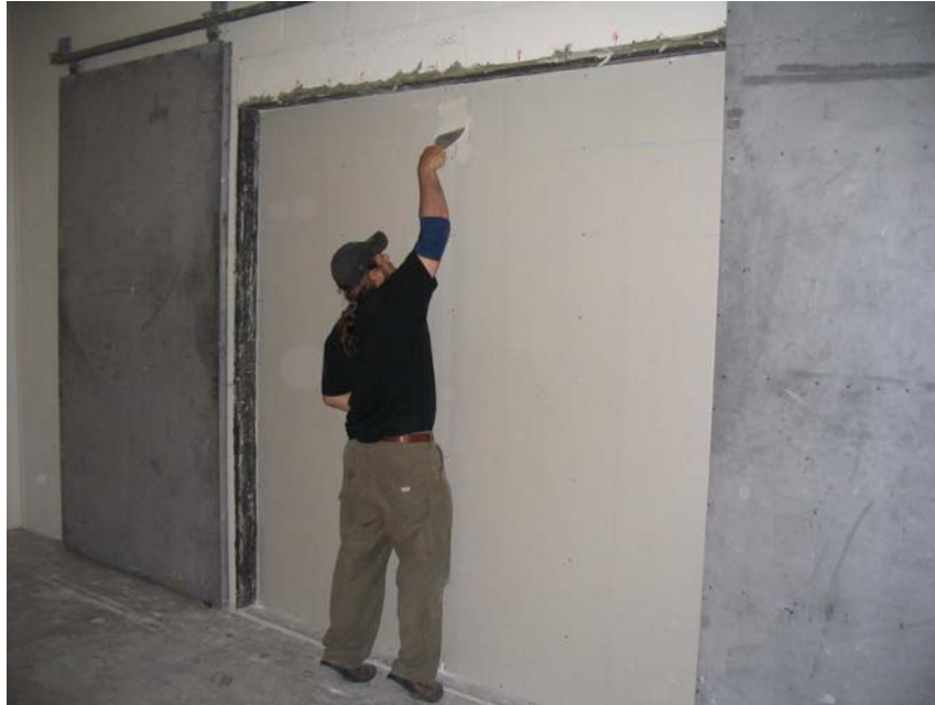
Figure 2: Mudding the center seam
