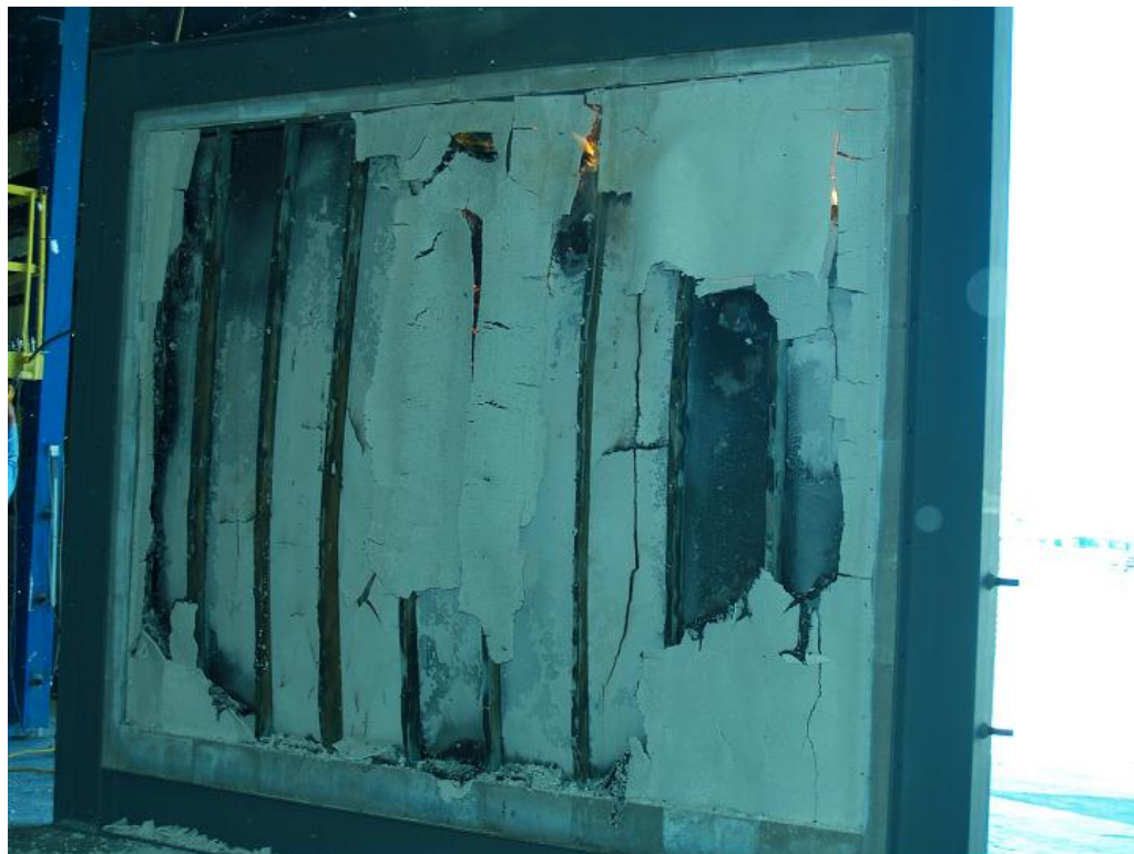
Figure B- 6. Exposed Face of Fire Test Wall at end of Furnace Exposure.
