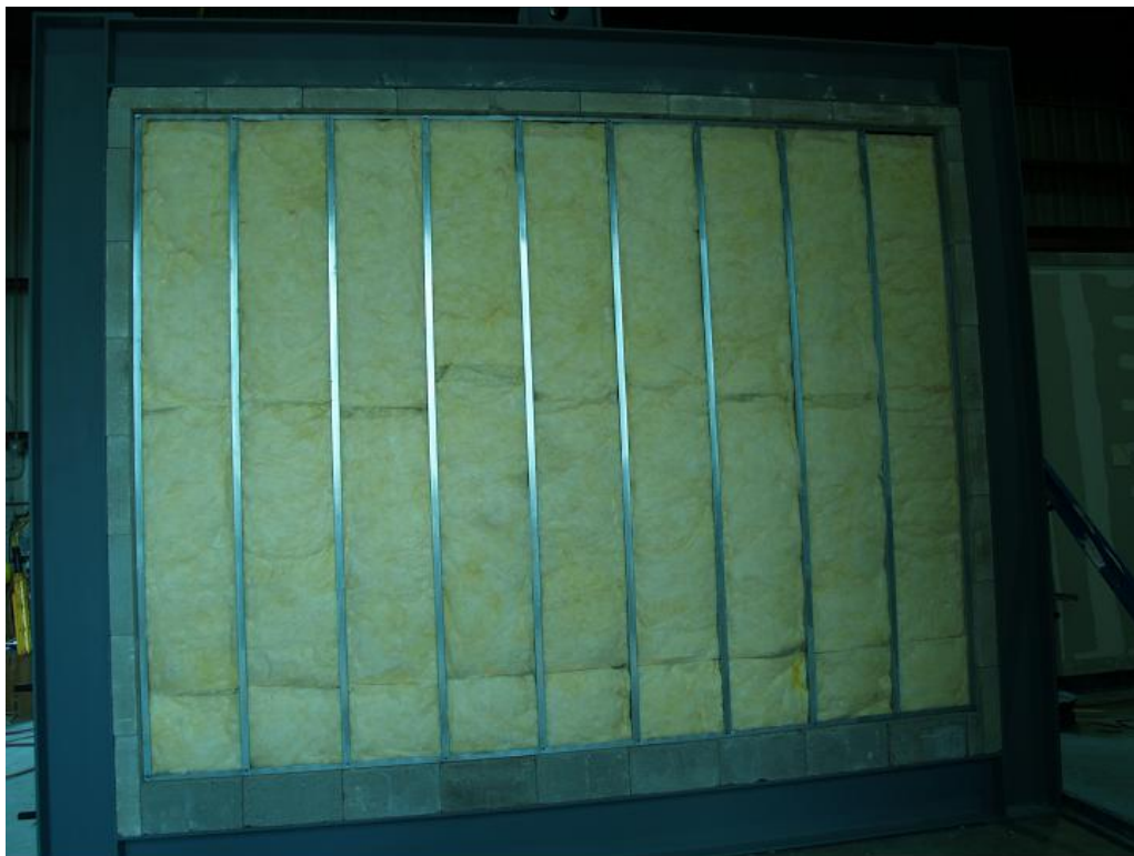
Figure B- 2. Test Wall during Construction.
