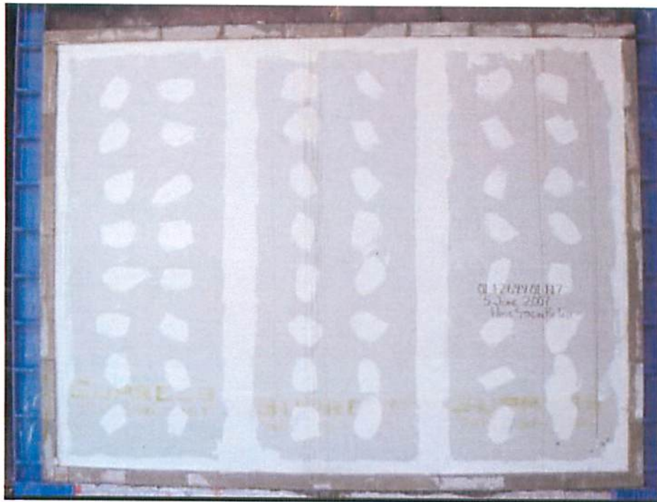
Figure A-9. Unexposed Side of Hose Stream Retest After Hose Stream Test.
